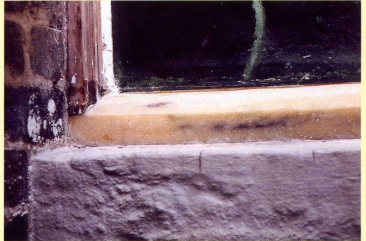
5. Repair completed with Dry Fix/Dry Flex RP.
