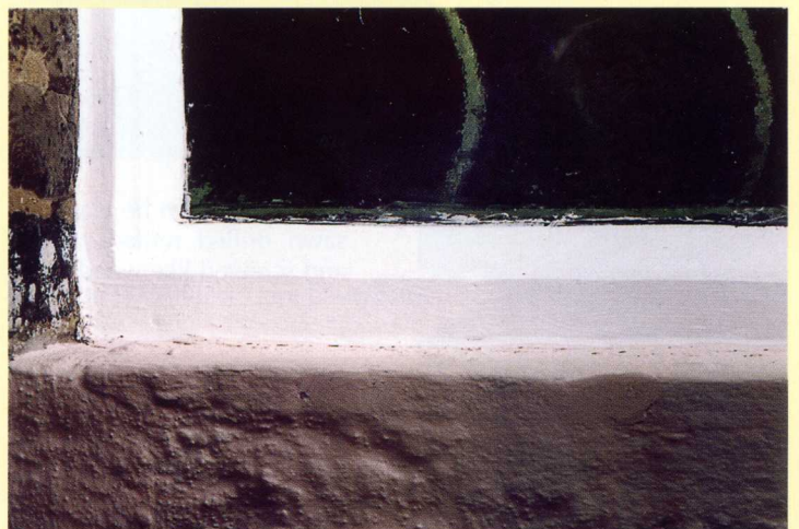
6. The repaired window is painted.
