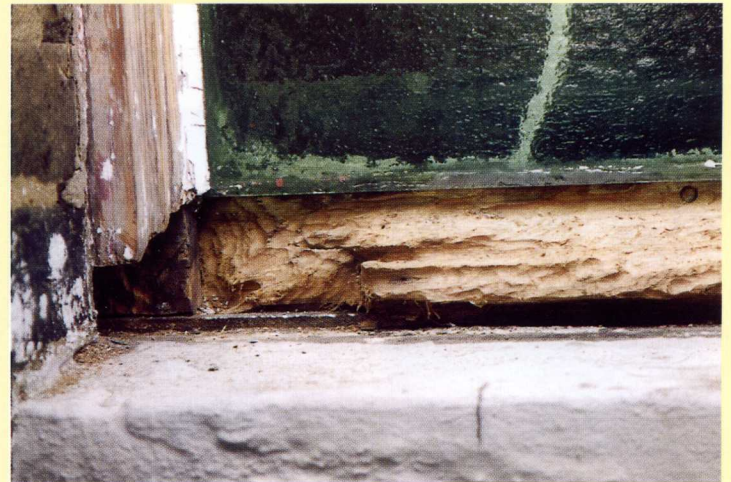
4. Wood decay removed with the Window Care Profi.
